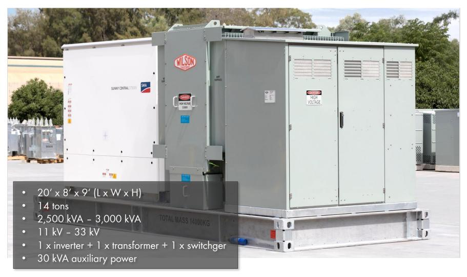
> Compact Solution for smaller PV Plants or to mix with 40' unit
