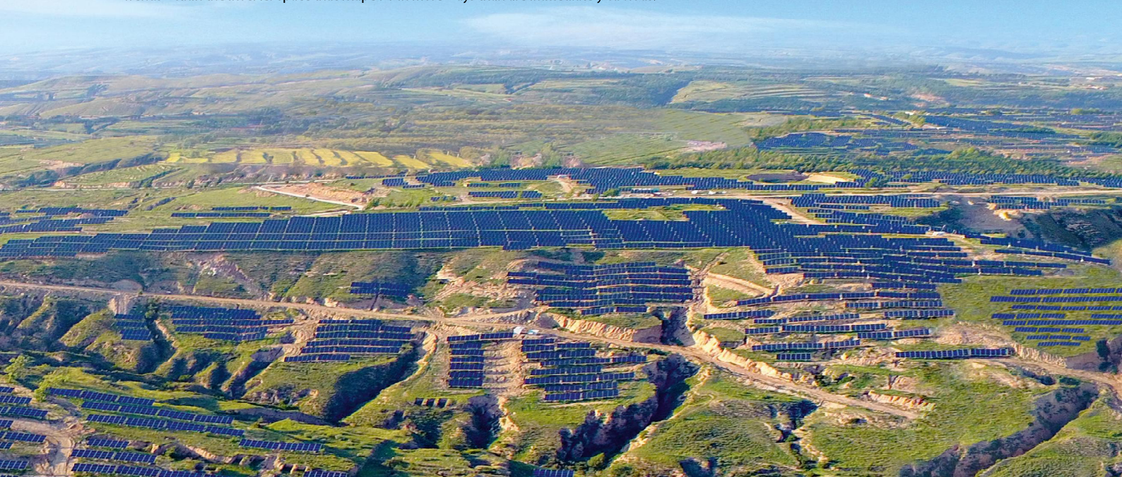
A sea of modules, controlled by string inverters: Such a sight is increasingly common across the globe. Trends within the inverter space that shape PV in more ways than are immediately obvious.
