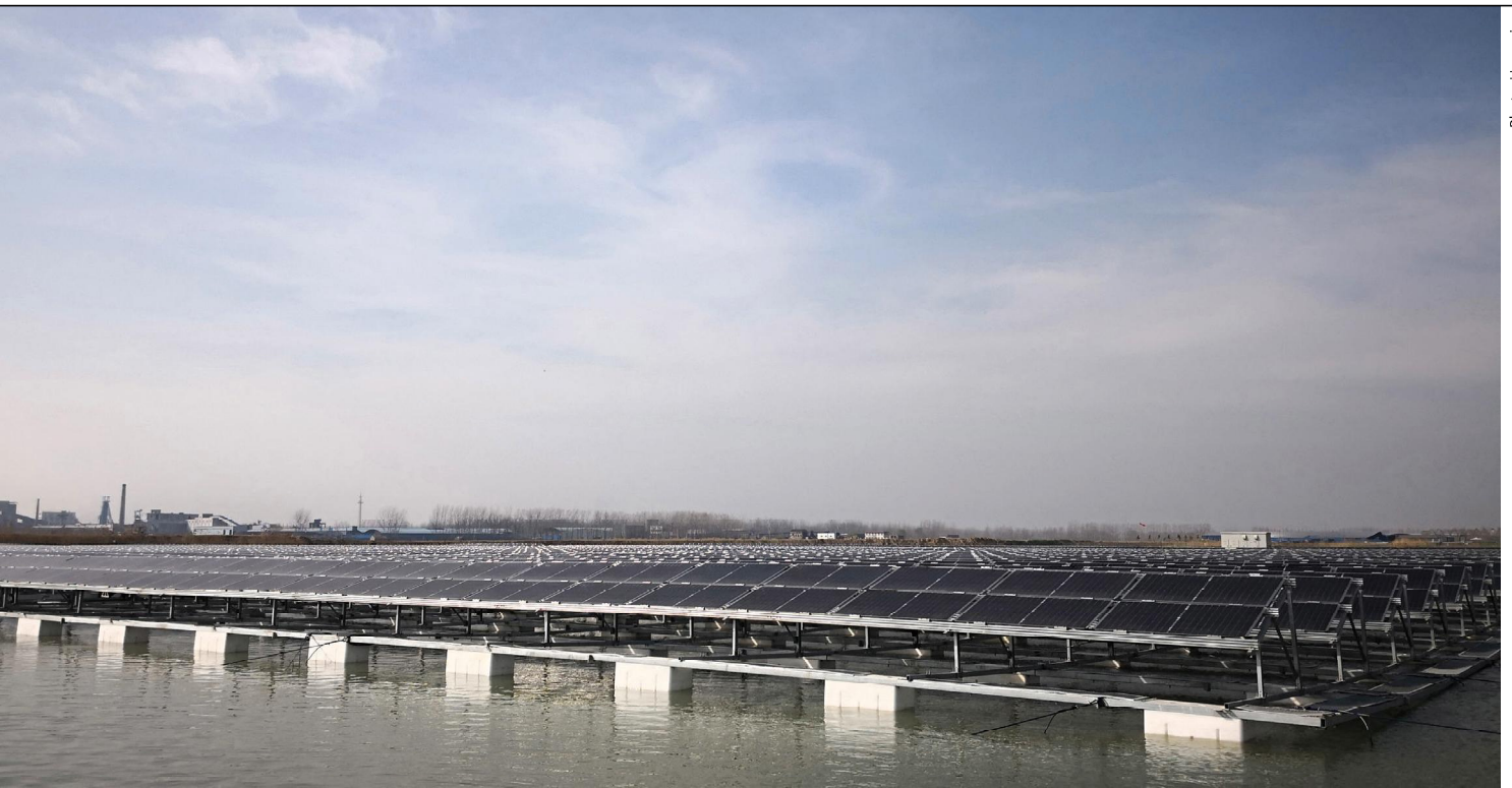
A PV project on water featuring bifacial modules and Huawei inverters. Depending on the surface albedo, bifacial modules can boost performance by between 5% and 39%.
