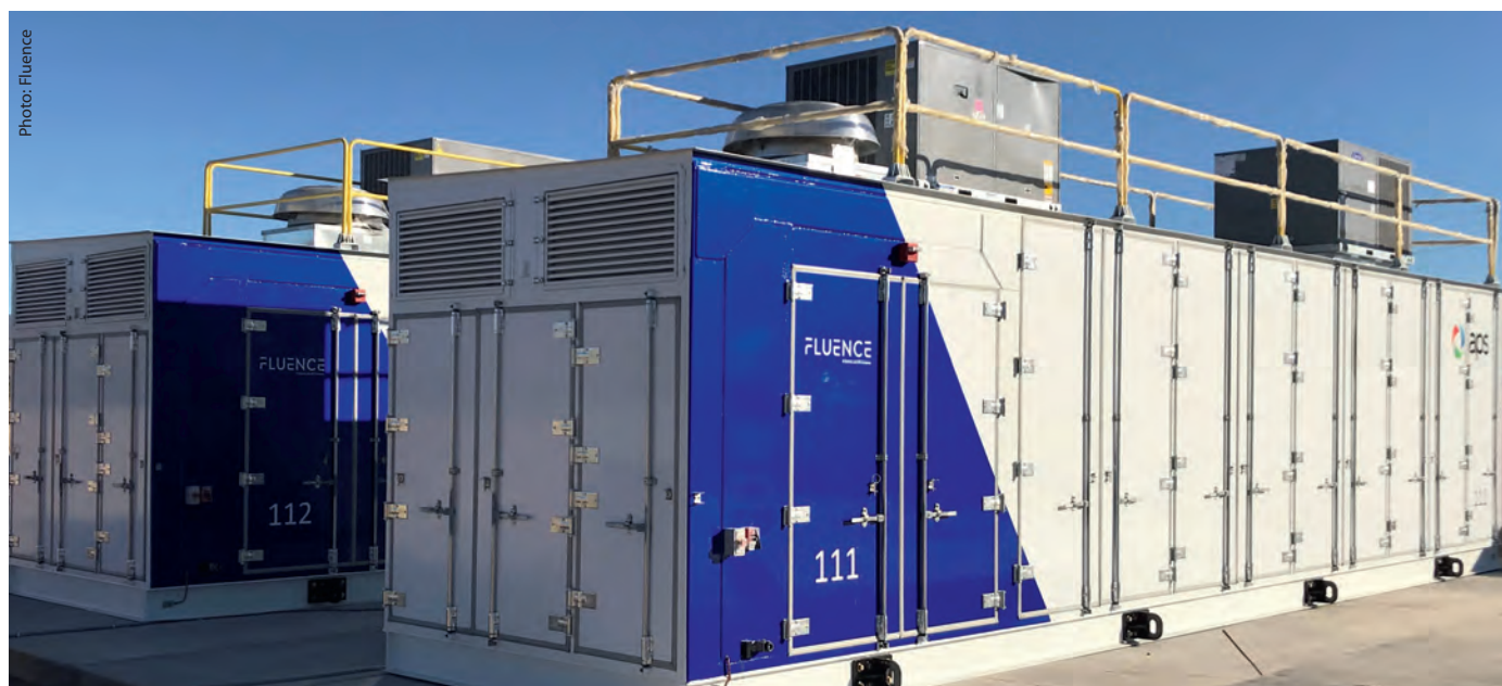
A 1 MW/ 4MWh storage system operated by utility Arizona Public Service in the town of Punkin Center.
