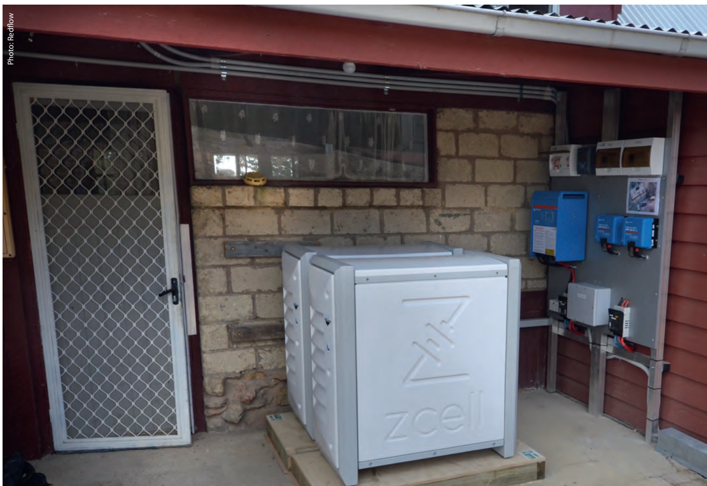
Australian manufacturer Redflow's Z Cell is a zinc bromine flow battery, and the first flow battery to be launched for residential purposes.
