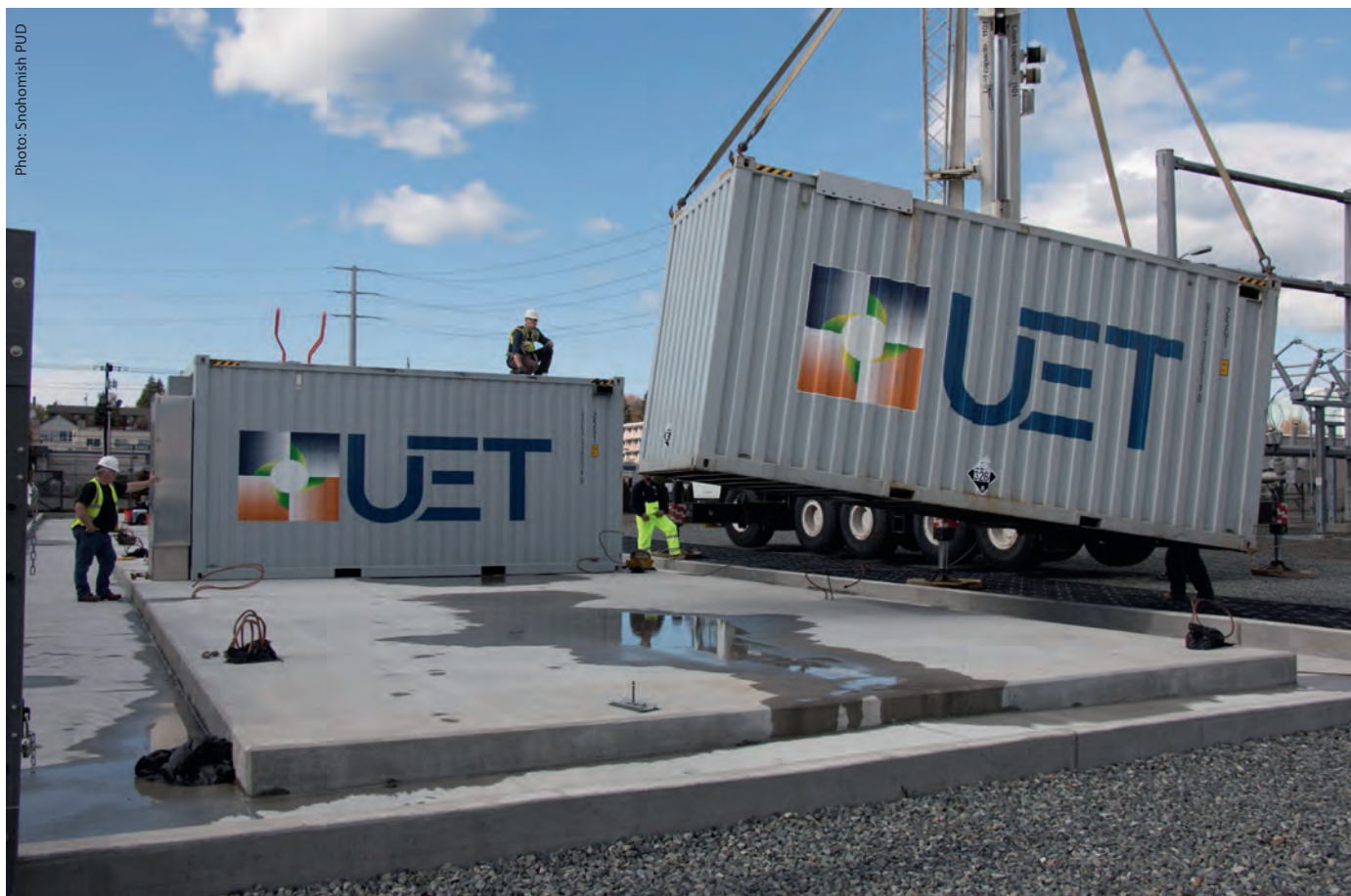
Unienergy Technologies' containerized 2 MW / 8 MWh Vanadium Flow Battery being installed in Snohomish County, Washington State, USA.
