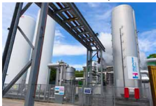
Highview Power's 5 MW pilot-scale cryogenic energy storage facility cools and liquefies air.
