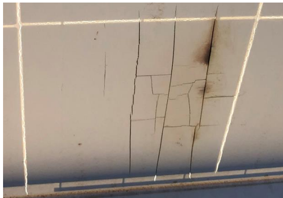
Overheating at cracks
