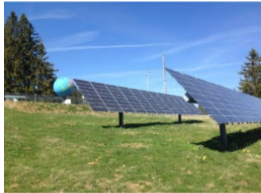
Mont Soleil, Switzerland 1992 0.3% annual degradation
