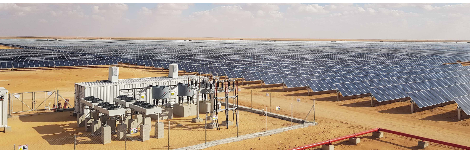
The 300 MW Sakaka Solar Plant incorporated TBEA's Static VAR Generators to support the grid, improve power quality, and save power.
