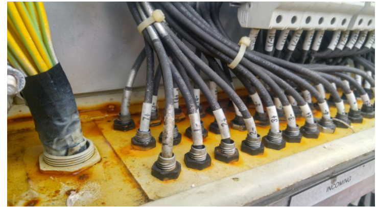
Water ingress and mild corrosion
