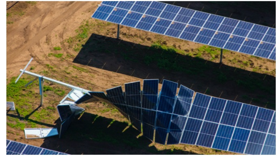
Twisted modules illustrate the damage incurred at the Oakey 2 site in October 2018.
