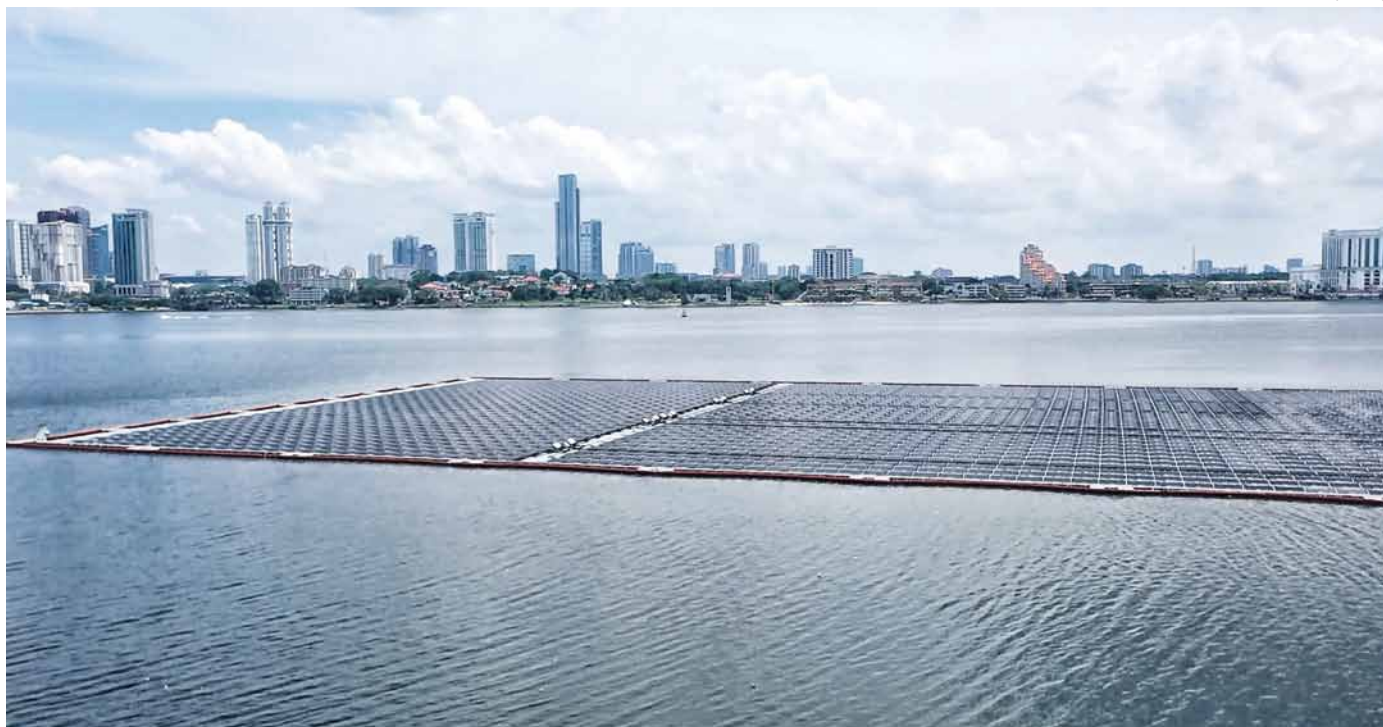
This 5 MW floating PV project in Singapore, developed by the Sunseap Group, powerfully demonstrates the effectiveness of such applications when executed with the right technology providers.
