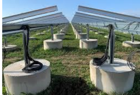
Embedded on concrete blocks
