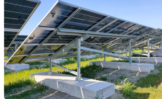
Screwed on concrete bases
