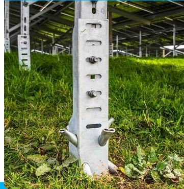
Embedded on concrete blocks
