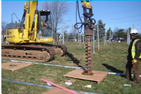
Pre-drilled holes + concrete/gravels
