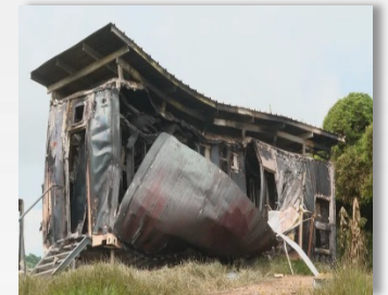
French box energy storage explosion accident in 2023
