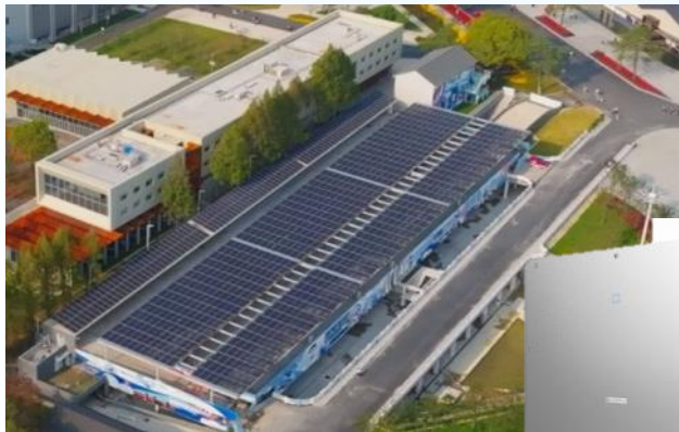
Commercial and Industry Roof
