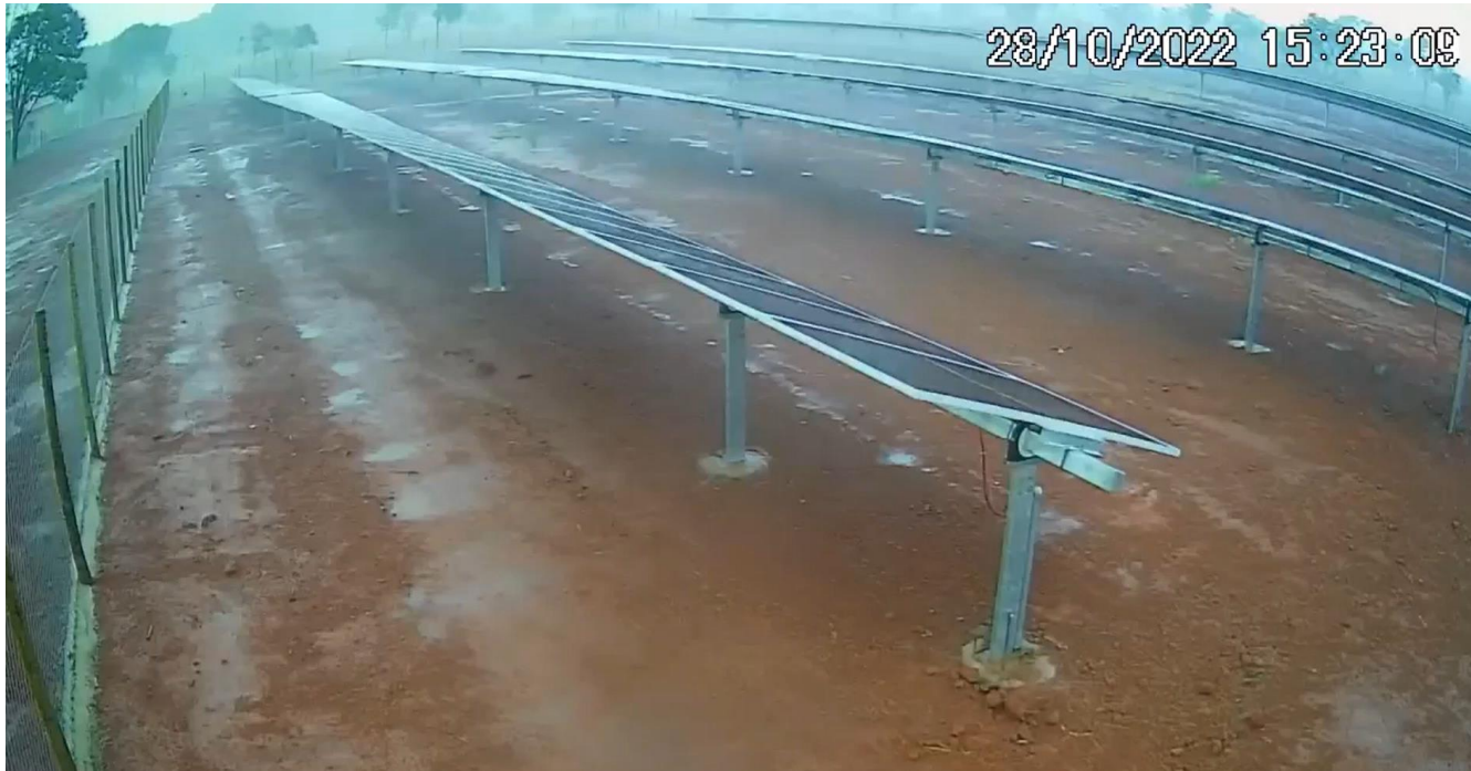
Video: Tracker array experiencing torsional instability (LinkedIn)
