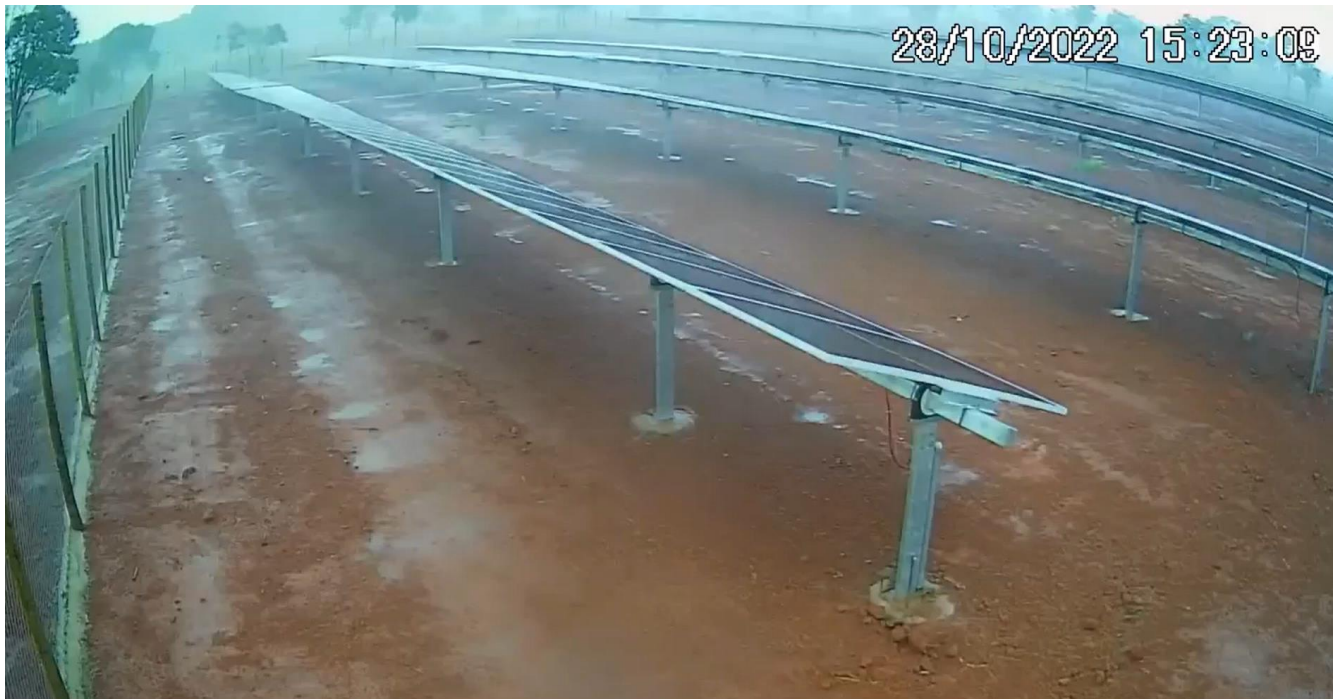
Video: Tracker array experiencing torsional instability (LinkedIn)
