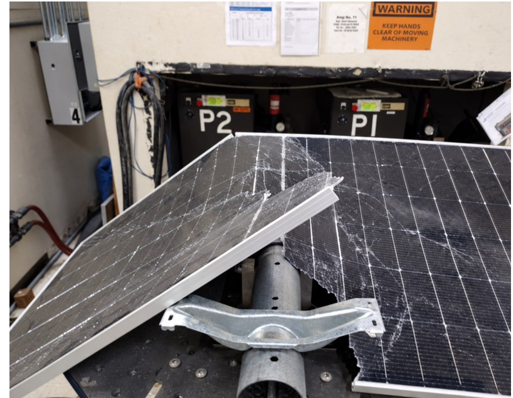
Frame Fatigue Failure
